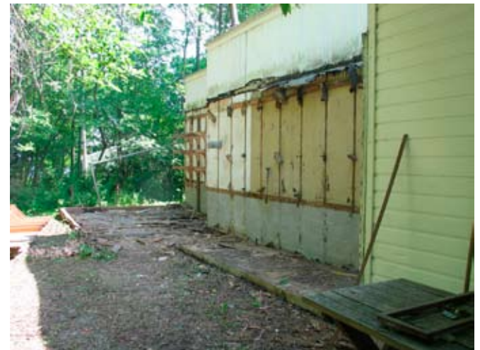
The lean-to sheds on the outside of the building were in disrepair (above) and needed to go. A volunteer crew made quick work of the project (below, after demolition). New windows will now be installed to allow light to enter the multi-purpose room being created inside the old “boathouse” section of the building. Photos by David Mathiason.
